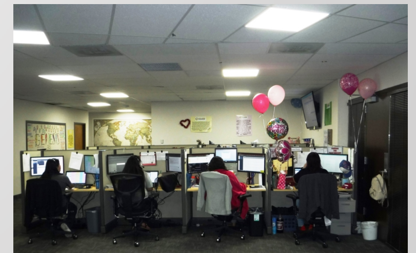
Figure 4 – New 2'x2' LED Fixtures
