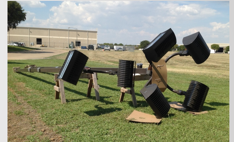
Figure 3 – New Pole and Lights
