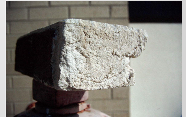
Figure 7 – Head joint of removed brick – typical.
