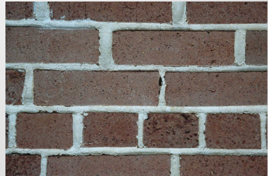
Figure 5 – Un-tooled joints in new wall.
