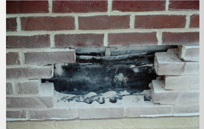
Figure 8 – Opening in the parapet wall
