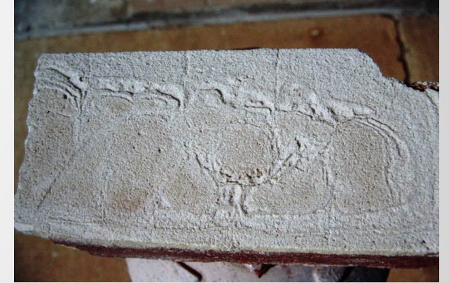
Figure 6 – Top of removed brick with mortar – typical.
