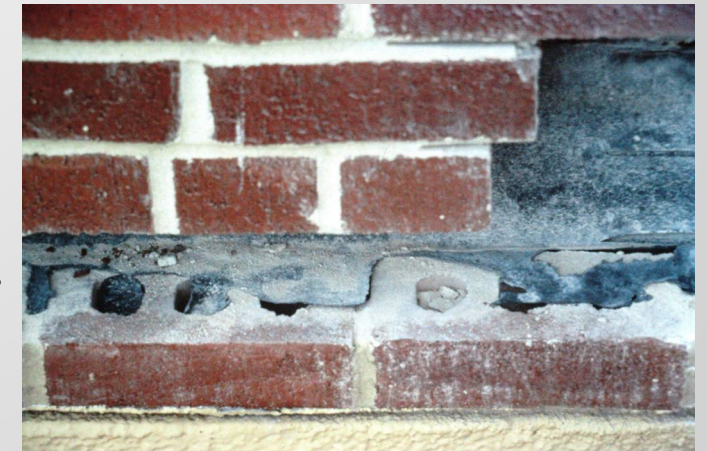
Figure 9 – Opening in the parapet wall
