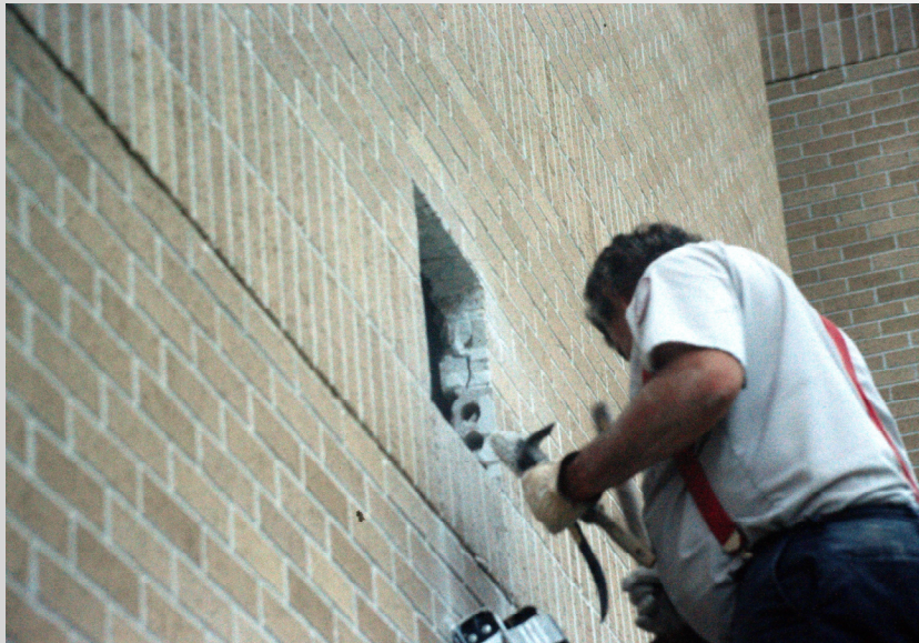
Figure 4 – Opening at the floor belt course.
