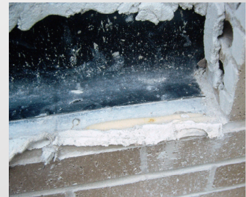
Figure 9 – Wall cavity at the belt course
