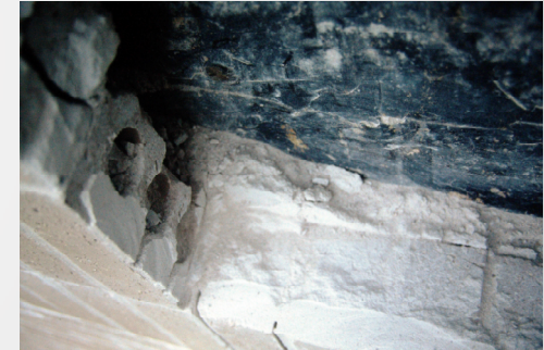
Figure 8 – Wall cavity at the belt course
