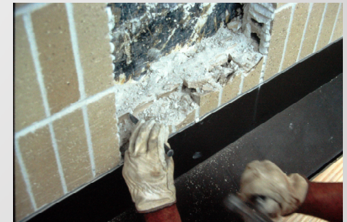
Figure 13 – Wall cavity at the belt course
