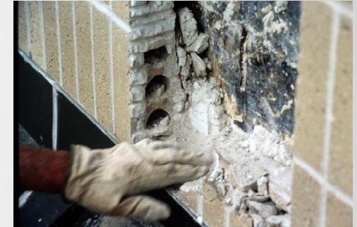
Figure 12 – Wall cavity at the belt course
