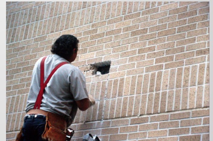
Figure 3 – Opening above the soldier course.
