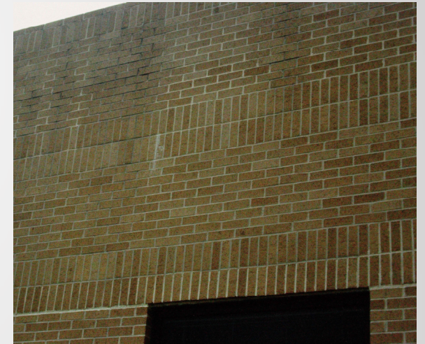
Figure 2 – Stains from water intrusion
