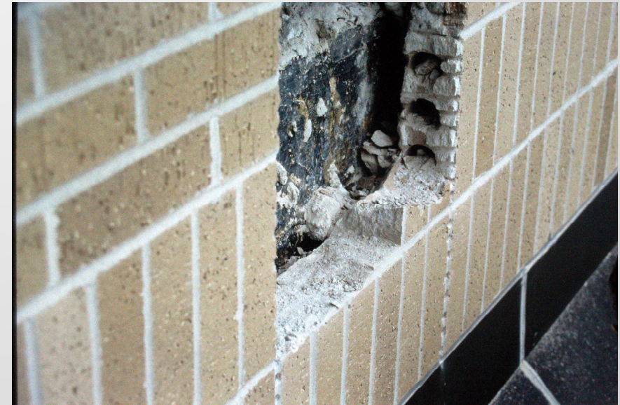
Figure 5 – Opening at the floor belt course.
