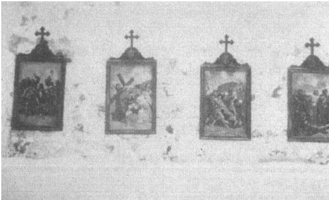
Figure 9 - Incorrect practice using a tight cement type plaster
