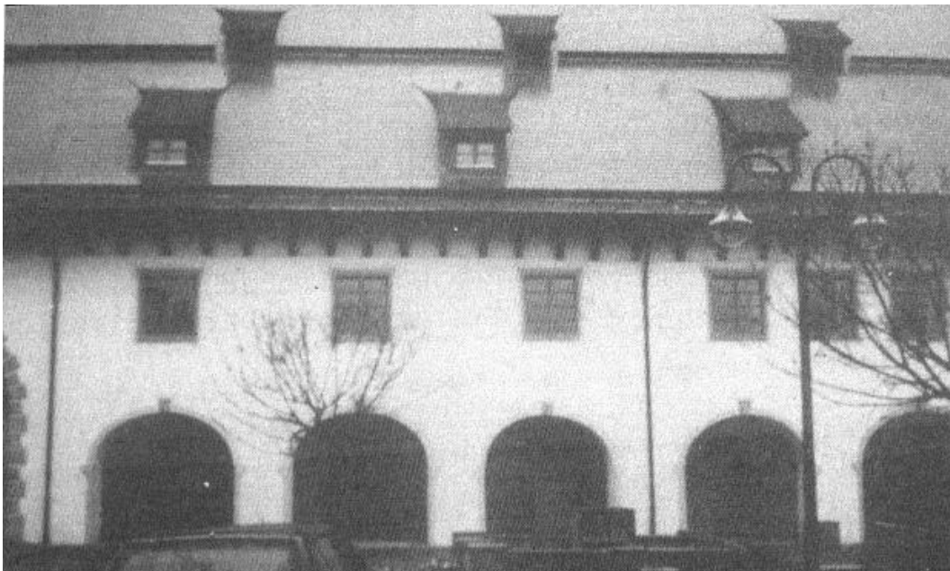
Figure 12 - Repair of the Monastery using re-development plaster
