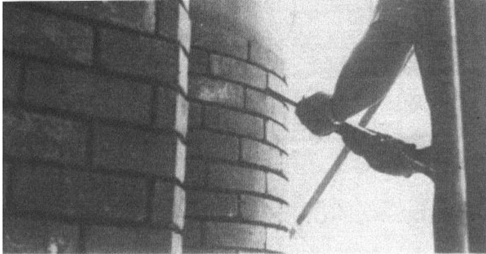
Figure 23 - Removing mortar with power chisel. Preparing the wall for tuckpointing phase
