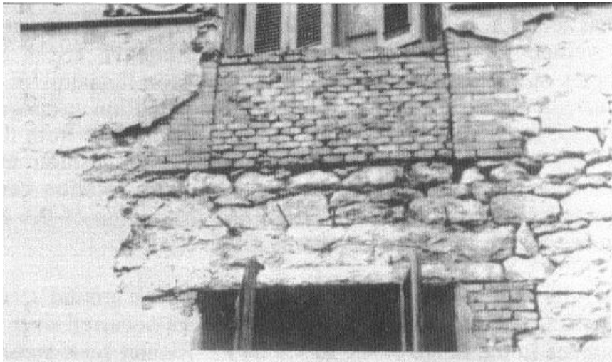
Figure 6 - Use of stone and brick masonry around window openings.
