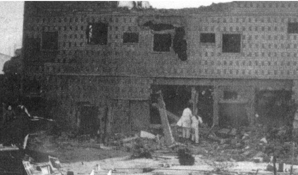
Figure 19 - Building with a RC frame, with infill masonry walls, subjected to shelling.
