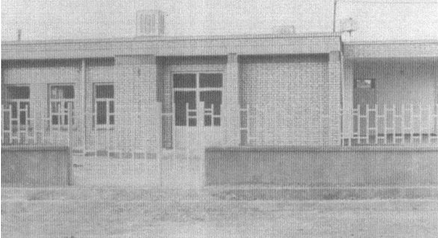
Figure 16 - Engineered reinforced masonry building that survived the Sirch earthquake of July 28, 1981.
