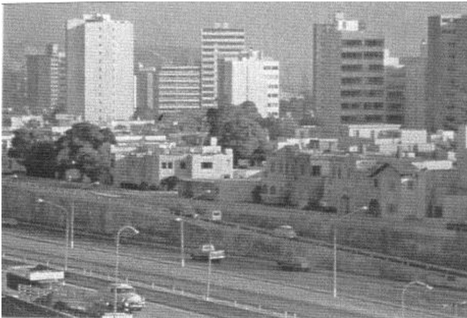
Figure 31 - Reinforced concrete and masonry high-rise construction in Lima. Low-rise reinforced masonry housing units in the foreground.
