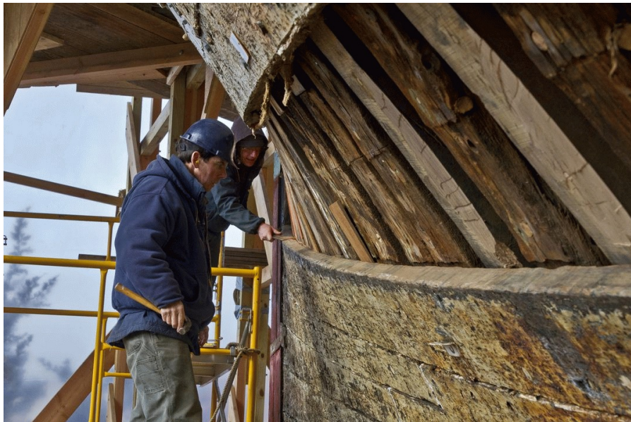
Figure 6 - Work on the exterior of the keel
