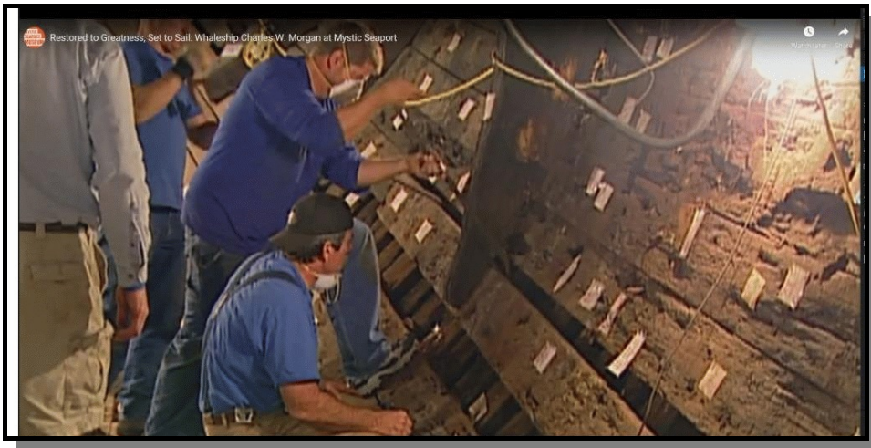
Figure 4b - Working on the interior of the hull.
